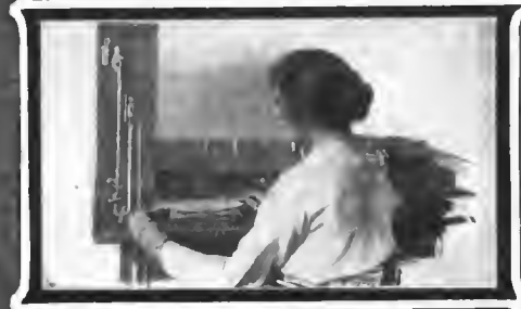
Testing the range of thermometer tubes for Boyce Moto-Meters.
